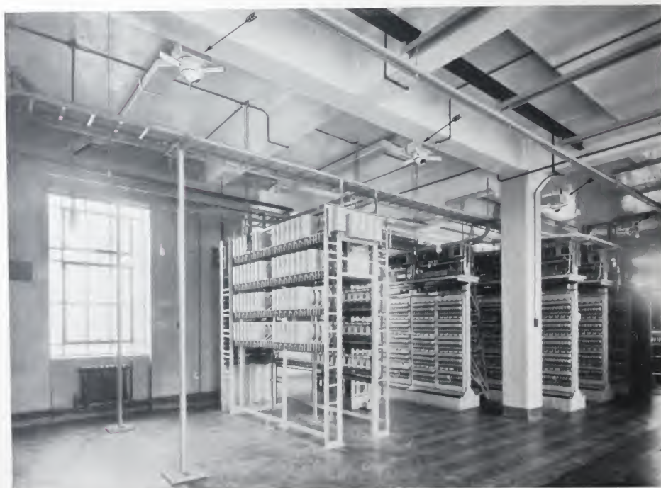
IN A TELEPHONE EXCHANGE
