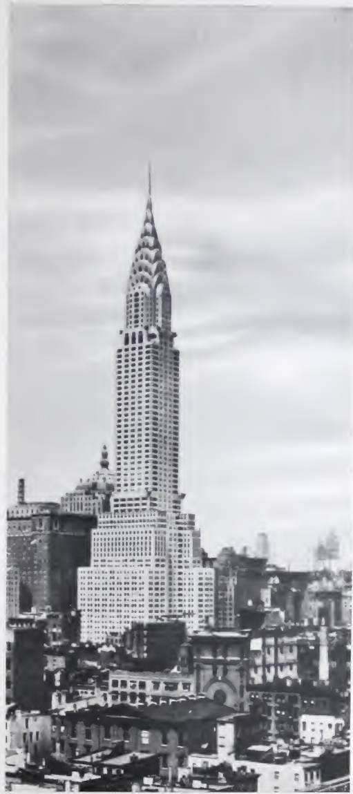
THE CHRYSLER BUILDING, NEW YORK THE WORLD'S TALLEST STRUCTURE 77 STORIES
