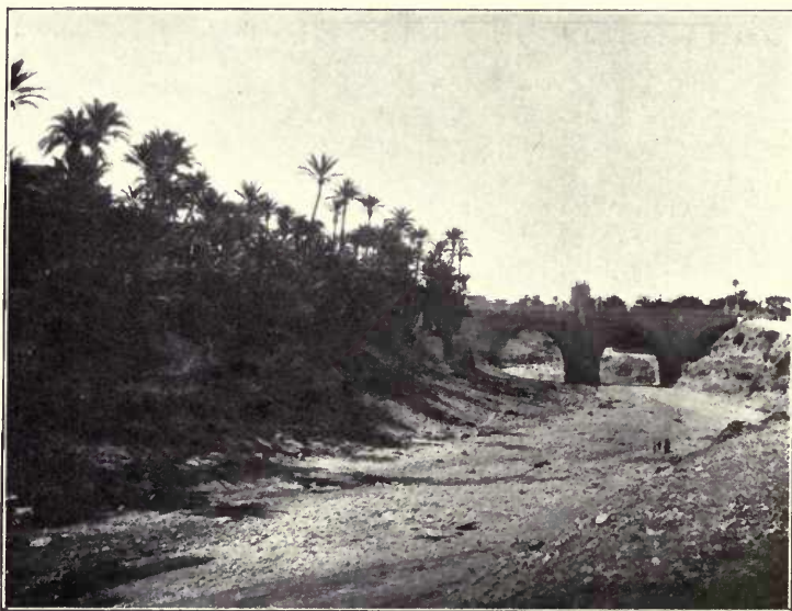
THE BRIDGE AT ELCHE.
